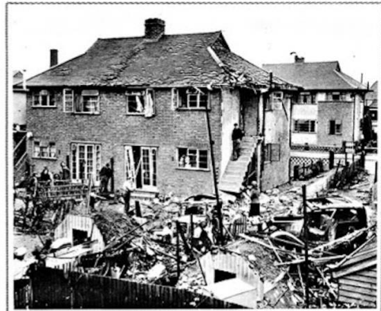
TWO ANDERSON SHELTERS IN THE SAME DISTRICT AS THAT SHOWN IN THE PHOTOGRAPH ON THE LEFT, ALSO INTACT. (Planet.)
