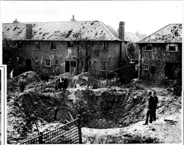
A LARGE BOMB-CRATER BEHIND A ROW OF DAMAGED HOUSES AFTER THE CROYDON RAID: THE SHELTERS WERE UNAFFECTED. (Keystone.)
