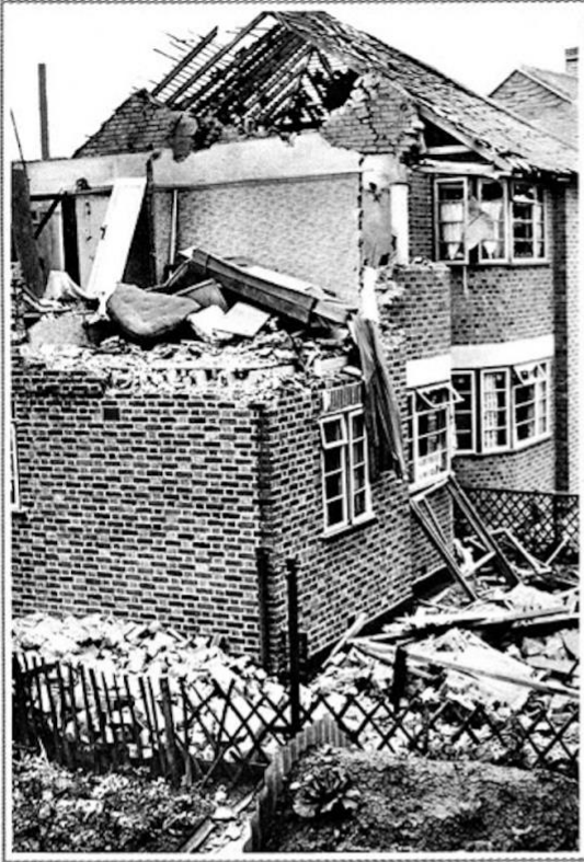
AN ANDERSON SHELTER, CORRECTLY COVERED WITH EARTH (FROM WHICH CABBAGES SPROUT), UNHARMED DESPITE SURROUNDING BOMB DAMAGE. Wide World.
