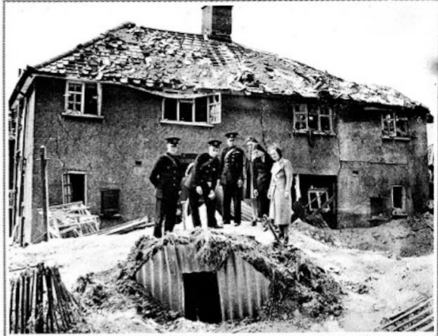
DAMAGED HOUSES, WITH AN UNTOUCHED ANDERSON SHELTER IN THE FOREGROUND, WHOSE OCCUPANTS FOUND COMPLETE SAFETY. (Planet.)
